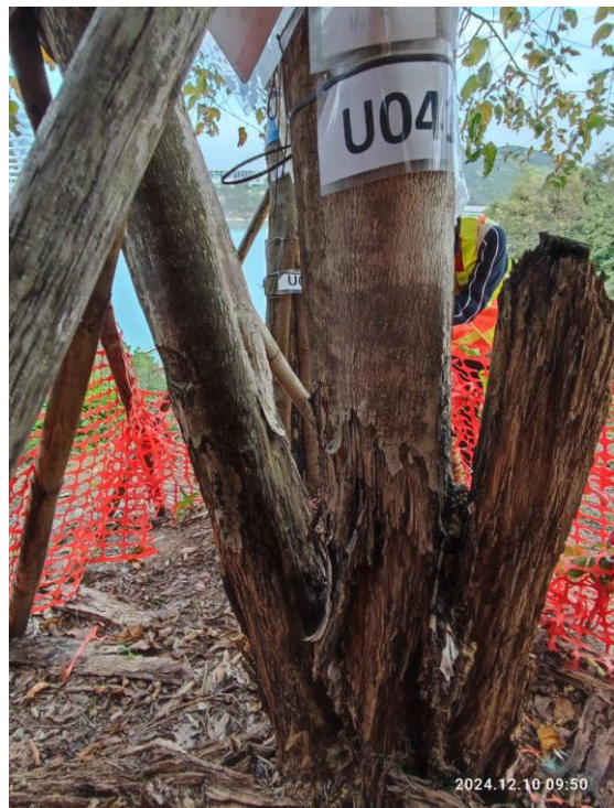
12: U041_Wood damage at trunk union#3
