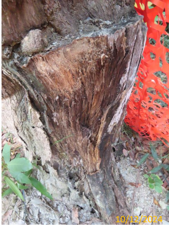
17: U043_Crack on trunk
